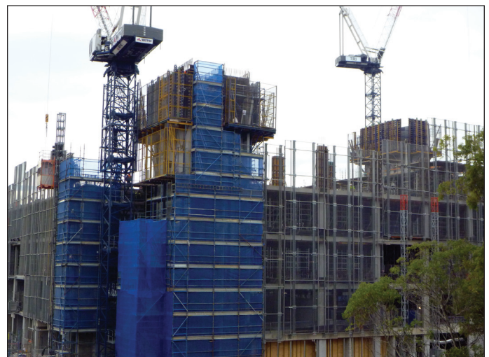
Figure 3. Construction of the Translational Research Institute Facility.
